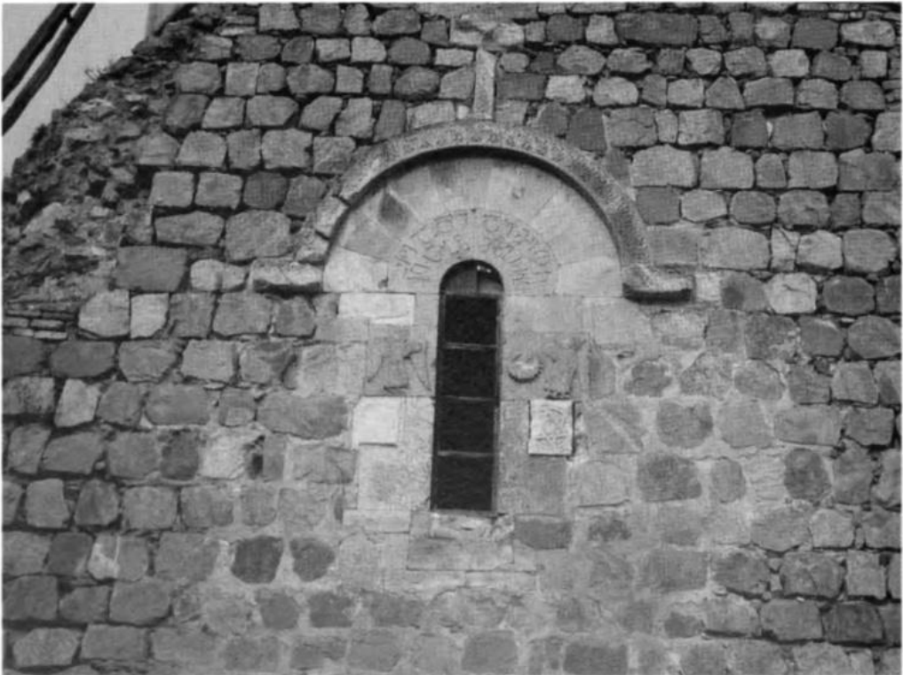
2. Mosque in Dolishan, former monastery church, south cross-arm façade
